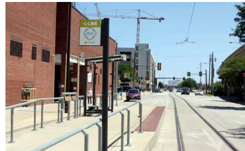
Track and catenary for the Lakeside loop are already in place at the future stop on Clybourn Street, looking east towards the unfinished development at The Couture.
